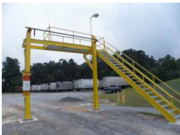
Fig. 1: Fixed tarping station for chips/residue shipping facilities.
